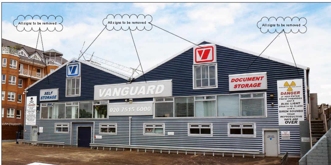
Figure 1 Existing Rear Elevation
