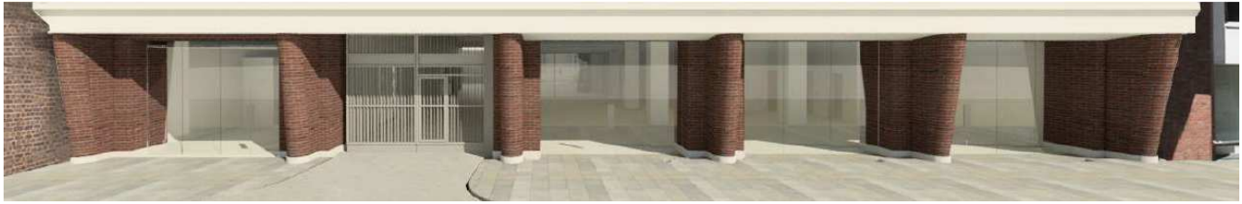
Existing Ground Floor Treatment
