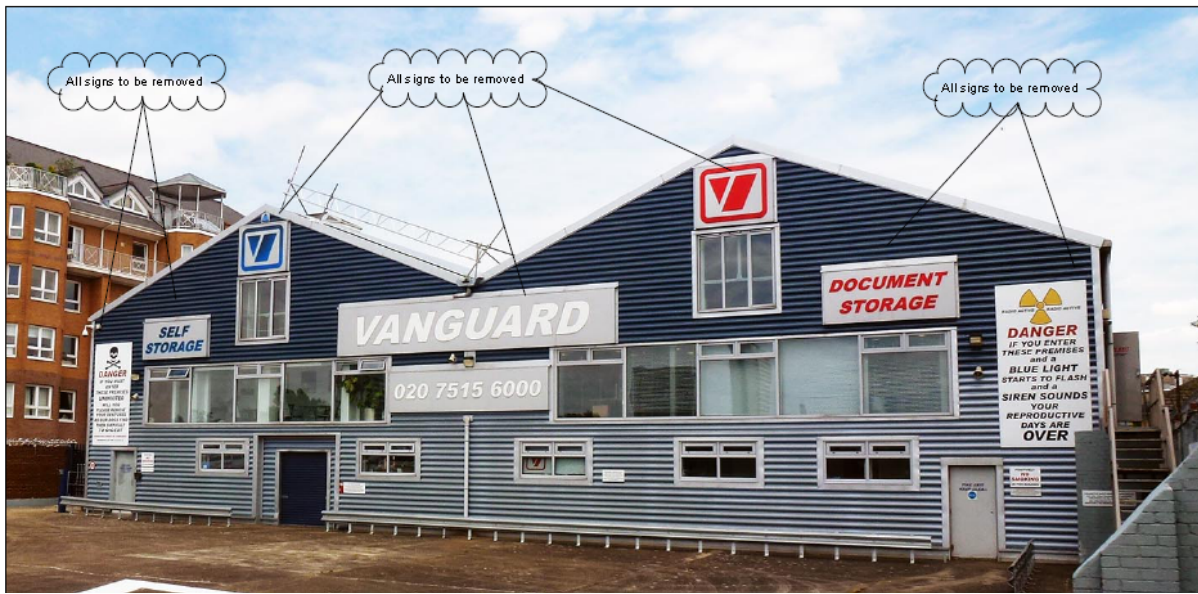
Figure 1 Existing Rear Elevation
